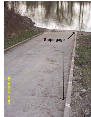
Figure B-51 – Reading the Profile (Slope) Gauge
