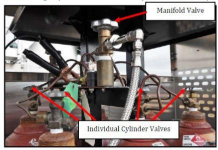
Figure K-5: AROS Manifold and Individual Cylinder Valves
