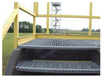
Figure K-13: Foot Plate at Top of Stairs
