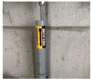
Figure K-9: Acceptable Markings for Helium/Hydrogen Tubing
