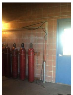
*Figure K-1: Properly Secured Cylinders (non-seismic area)*
